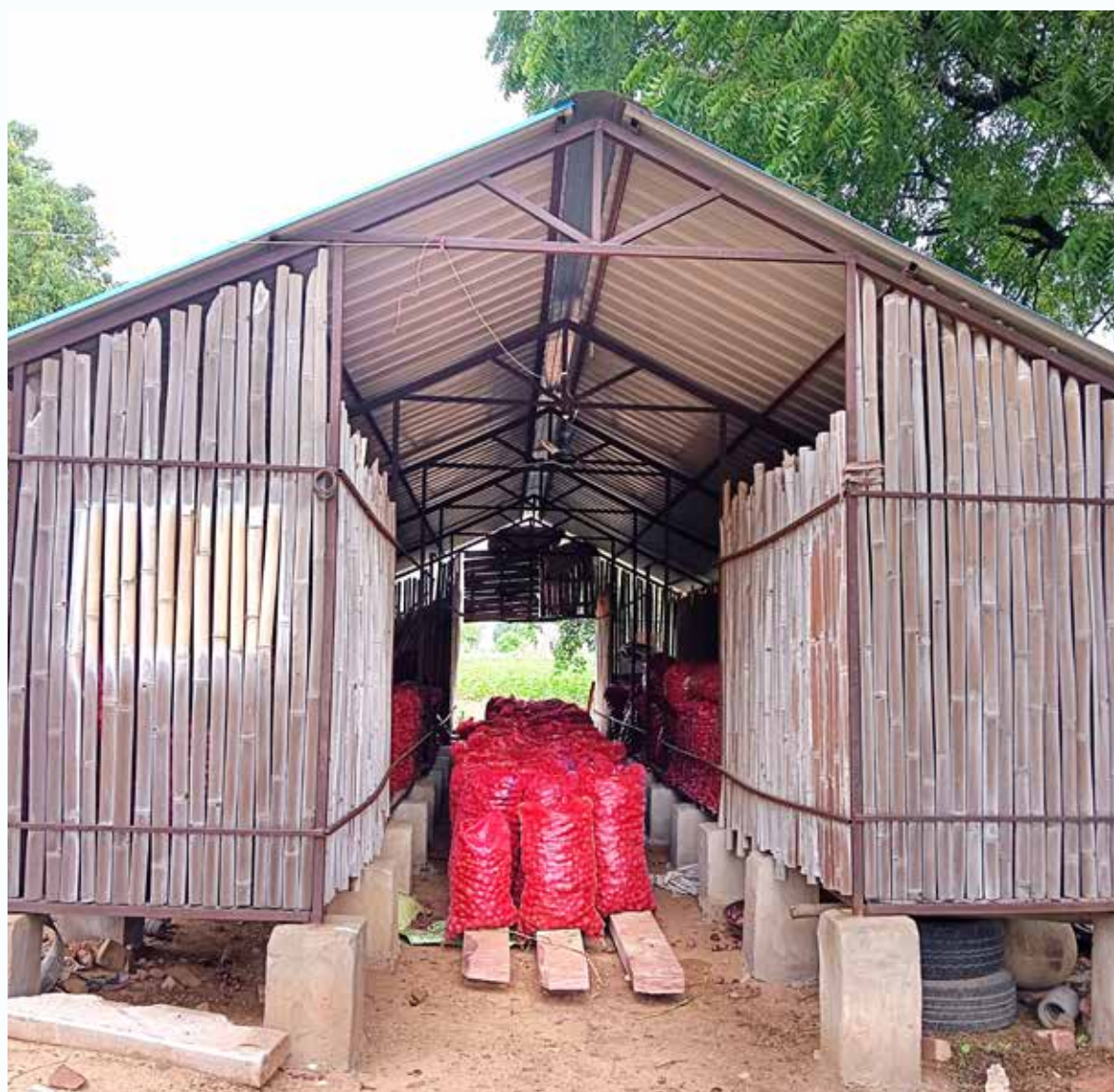
View of bamboo ventilated storage structure
