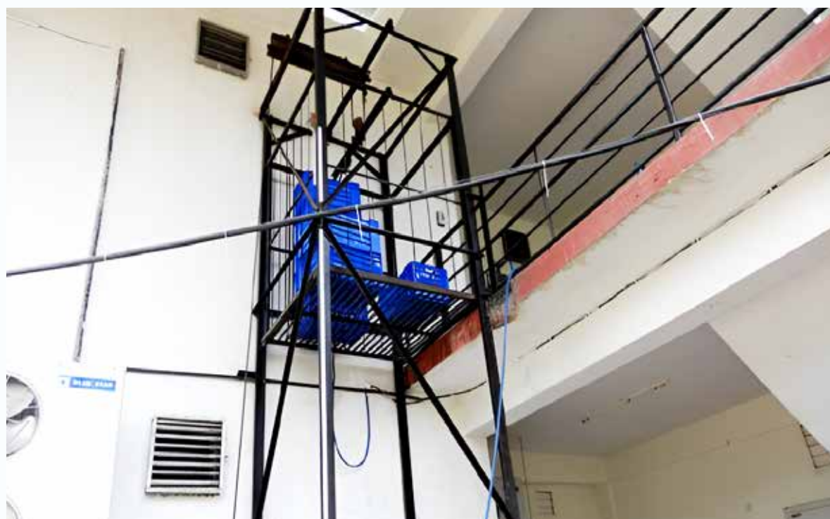
View of fabricated power lift
