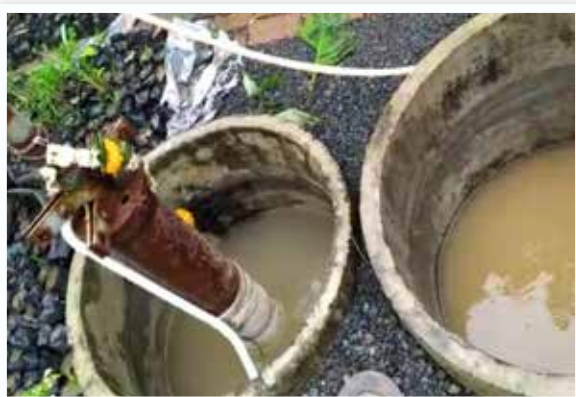
A view of bore well recharge
