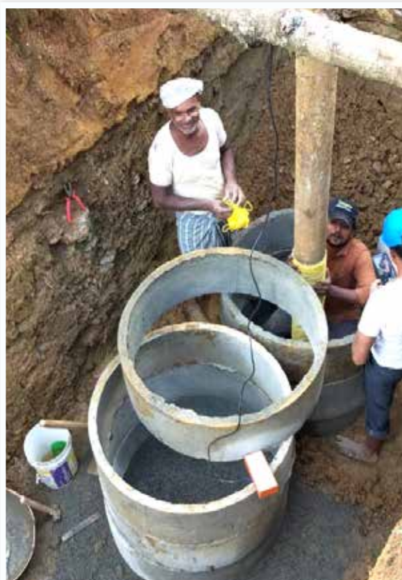
Development of twin ring method for recharging
