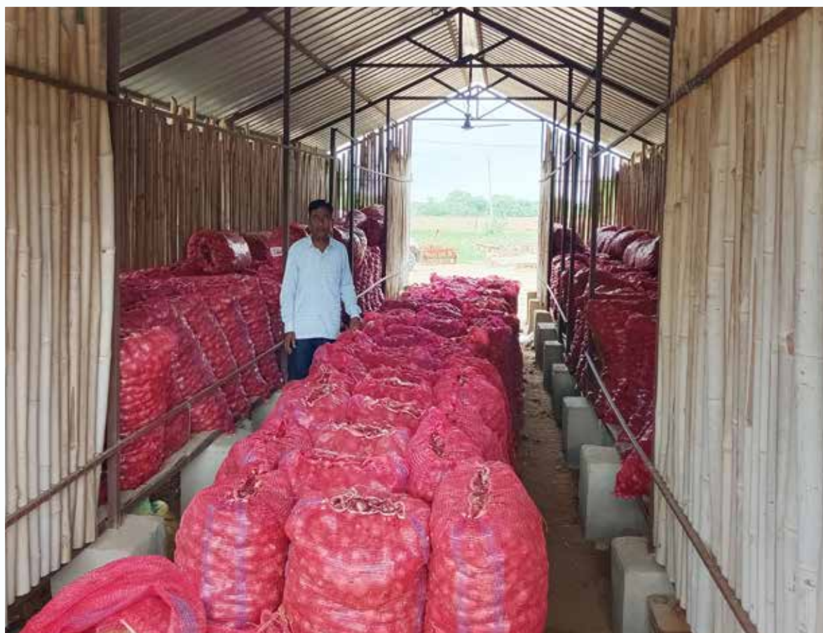
Santosh Kumar with bamboo-framed ventilated storage house
