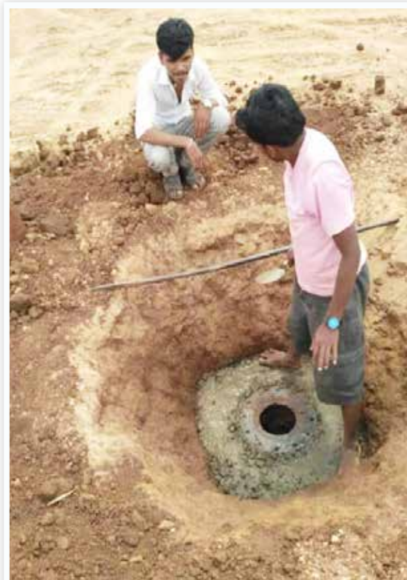
Development of twin ring method for recharging
