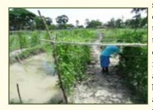
season. A peripheral canal is dug out and the earth is added to the existing land embankment to raise it upto 3 feet height and broaden to 5 feet bottom width. On an average 5-10% of the total land thus could
