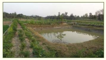
These derelict ponds were re-excavated and renovated upto a depth of 3ft. more over the existing average depth of 5ft. Proper embankment, inlets and outlets were also made. A portion of the silt was used to spread over the adjoining low lying agricultural field.
