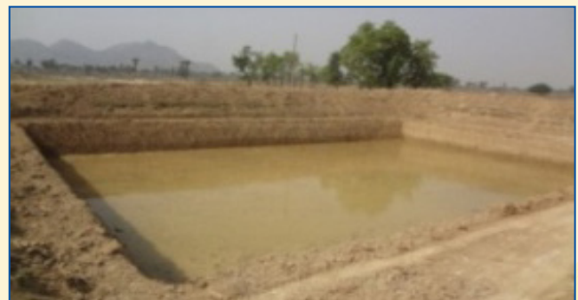
New Pond excavated
