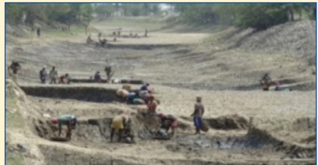
Renovation of canal
