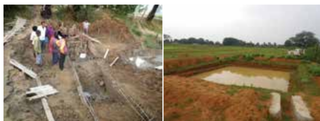
Check dam construction
