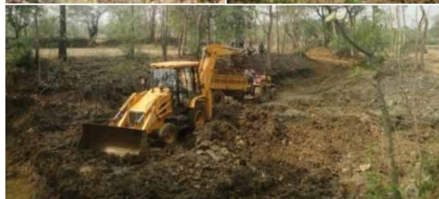
Before and after De-silting of channel
