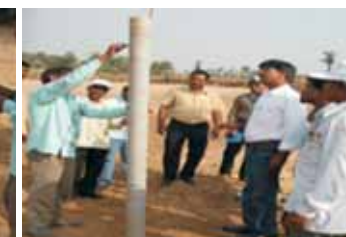
Perforated pipe inserted to lift water
