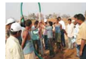
Connecting delivery &amp; perforated pipe
