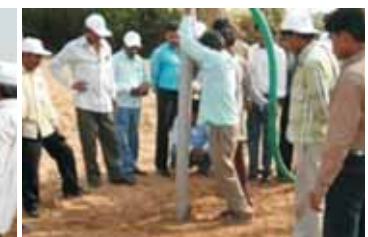
Inserting perforated pipe mechanically
